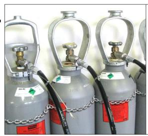
Place the CO2 bottles (liquid CO2 with dip pipe) on an even and solid surface. Place the bottles in such a position that the valve opening does not point in the direction of persons or objects. Place the CO2 bottles preferably outdoors or in a properly ventilated space with a CO2 detection system. CO2 bottles are pressure containers. That is why you must secure them with special gas bottle brackets or chains to prevent them falling over.
